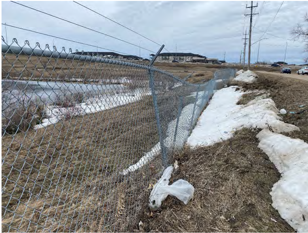
Photo 03: Instability located on the south side of Retention Pond 4-12, adjacent to Callsbeck Ave.
