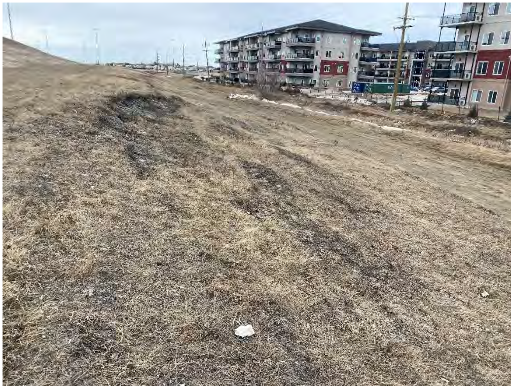
Photo 02: Shallow instabilities located on the lower east side of the south embankment.
