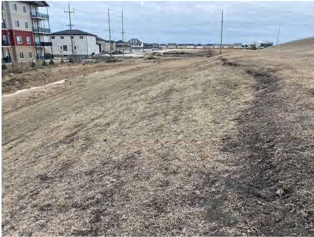
Photo 01: Shallow instabilities located on the lower east side of the south embankment.
